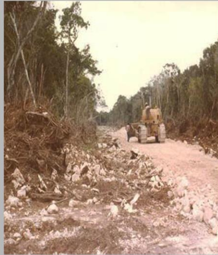
Roadwork Cozumel, Quintana Roo
