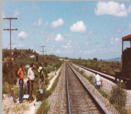
Civil Works "Mexico-Queretaro" Railroad
