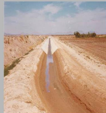
Irrigation Canal Guasave, Sinaloa
