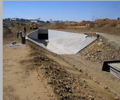
Civil Works Talamantes River
