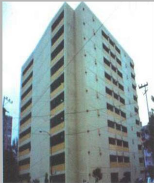
Somex Building Mexico City
