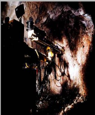
Ramp "San Alvar" Drilling Zacatecas
