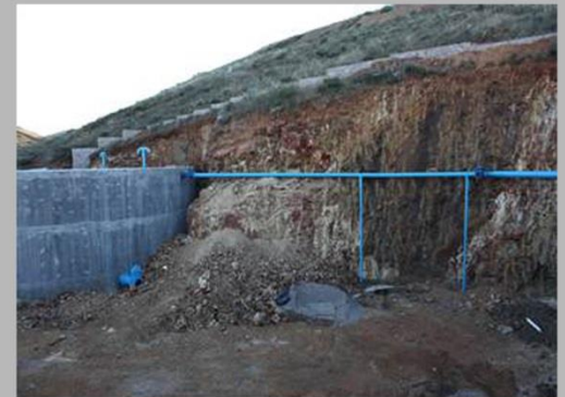
Infraestructura (Agua Potable)
